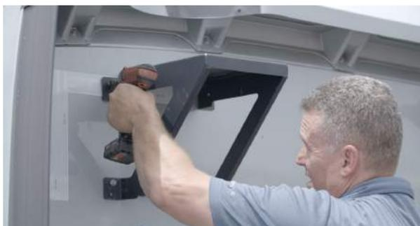
**7.** After all the Riv-nuts are secure, replace the Fixed Mount Base. Beginning on one corner of the bracket, start to hand tighten the 1/4-20 bolts with a couple of threads, then go back over, using the impact gun with a 7/16" socket, securely locking down all bolts.
