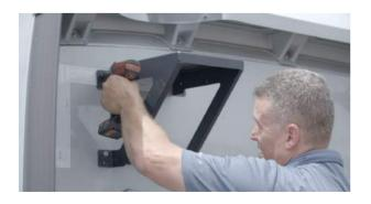
7. After all the Riv-nuts are secure, replace the Fixed Mount Base. Beginning on one corner of the bracket, start to hand tighten the 1/4-20 bolts with a couple of threads, then go back over, using the impact gun with a 7/16" socket, securely locking down all holts.
