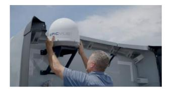
8. Now it's time to put the EpicVue satellite dome on the bracket. There are multiple sets of mounting holes on the Top Pivot Plate. Use the set of holes that allows you to get the dome as close to the truck as possible. Fairing extensions or other obstacles may necessitate using the outer set of holes.
