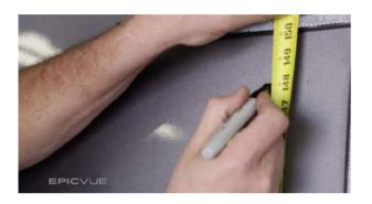
1. Make sure the mount is level with the top of the bracket measuring 12'4" off the ground. This will keep the dome, when secured to the mount, high enough to receive signal but lower than the required DOT height restriction of 13'6". Begin by measuring 12'4" from the ground and making a mark on your sleeper.
